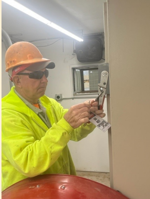
Monty Pearson is locking out a log washer and adding a "DO NOT OPERATE" tag prior to the maintenance.
